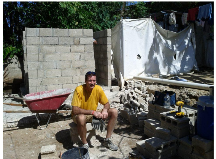
Finished with a pile of brick left – very, very tiring work.
