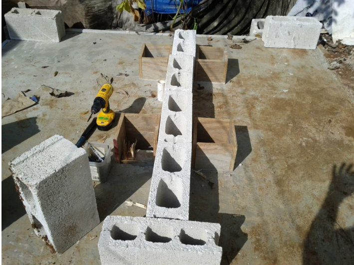
Next project, outdoor 4-stall restroom at orphanage.
