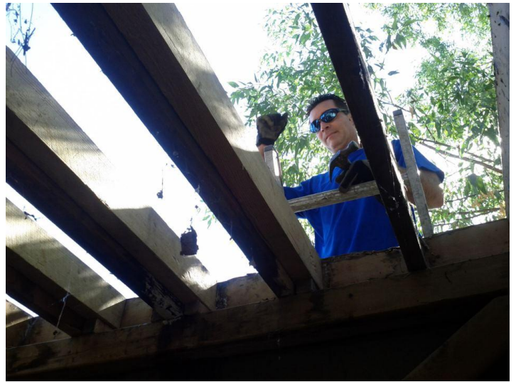
200 gal. water tank removed, now rebuilding wood base.
